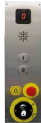
Lock switch IN-OUT to disable commands and light curtains (exclusive use for goods only transport)
